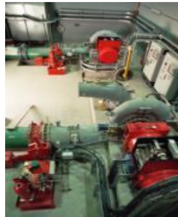
Photo 14. Two Francis turbine set on the treated wastewaters of Amman City, As Samra plants (Jordan) ( H = 42 m, Q = 2 \times 2.3 m 3 /s, P = 2 \times 807 kW, E = 8.6 GWh/year, 2007).
