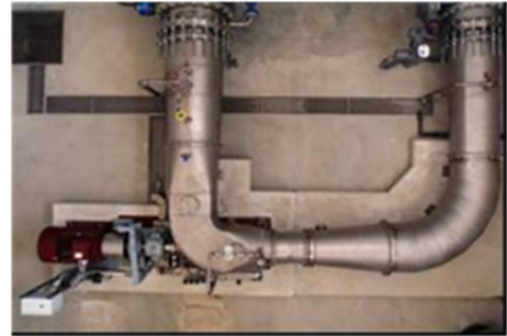
Fig. 7 and Photo 34. Setting of a Kaplan turbine as a bypass of an existing valve in a drinking water network (case study Poggio Cuculo).
