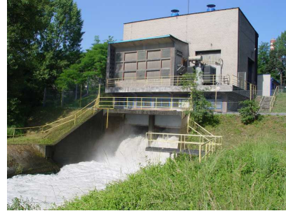
Photo 24. Skawina: the powerhouse during turbine overhaul.
