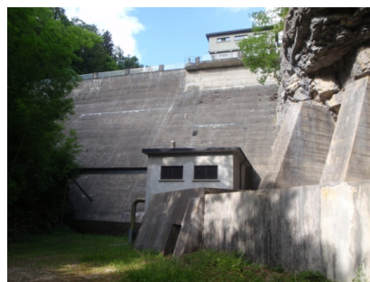
Photo 16. Le Day: The foot of the dam where the small power plant will be set.
