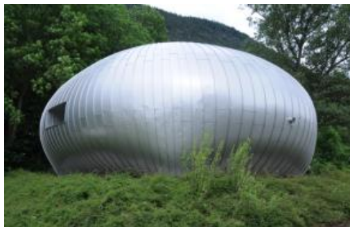
Photo 9. Seefeld: the power house.
