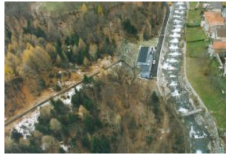
Photo 6. Rino: a view of the power station.
