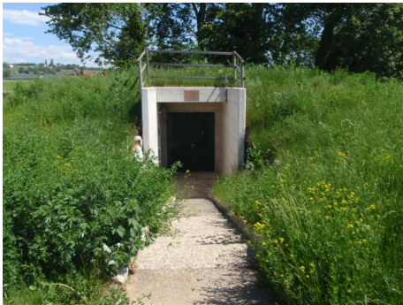
Photo 3. Armyary: the power house.
